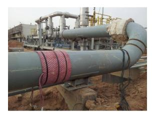
the heat affected zone of the metals and also increase ductility in these sections.
